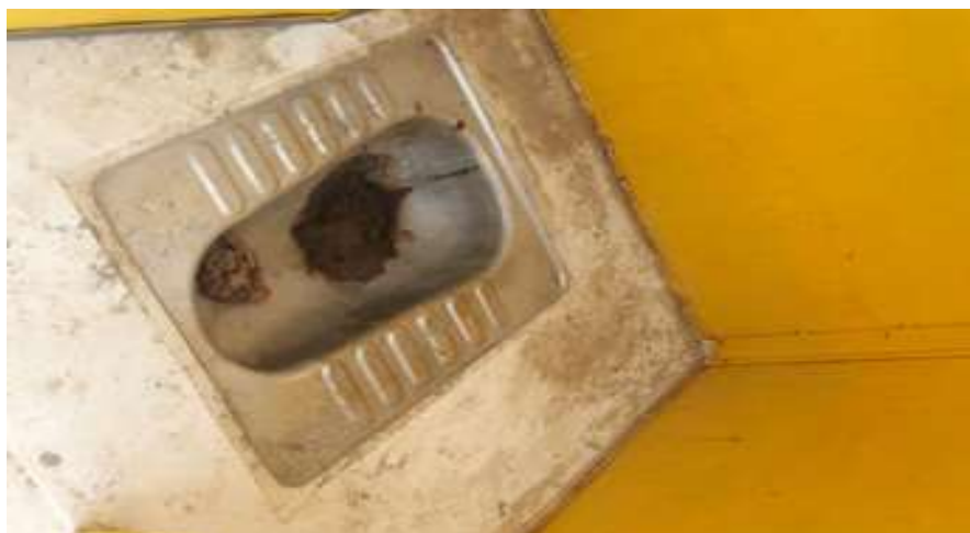
Photo: Condition of mobile toilets at Shahjahanpur
